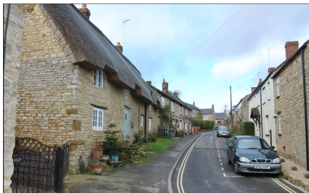
View of Mill Lane showing a mix of local building materials
