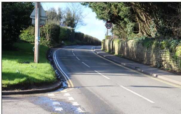
Bridge Road leaving the village towards Shutlanger
