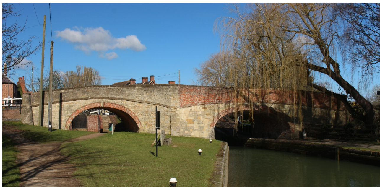
Canal Bridge built with local stone and bricks.
